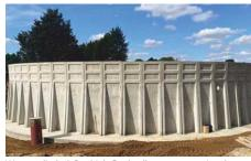
We supplied 4.3m high Sealwall precast sectional tank units to a waste water project in Norfolk
