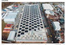
We completed a third solar panel installation - 1750 m<sup>2</sup> of panels at Wombwell, capable of generating up to 1180kwh of electricity/day. This- combined with previous installations at Cawthorne & Barugh Green gives us a combined total of 0.7 megawatts of on-site renewable energy capability
